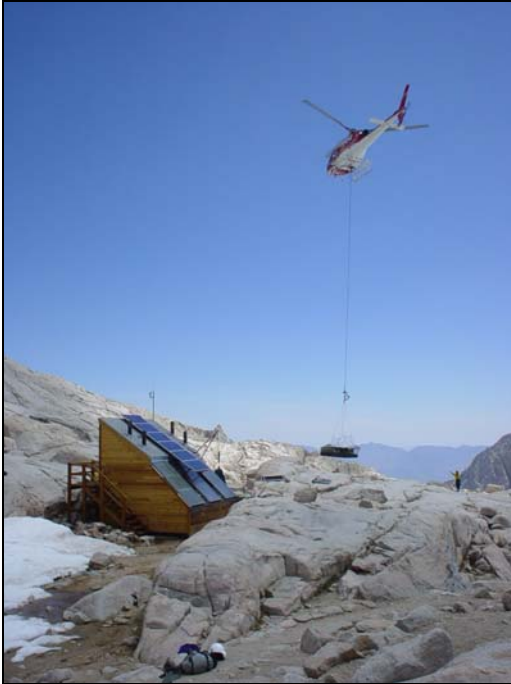
FIGURE 2: Helicopter performing maintenance at Trail Camp Toilet Facility
